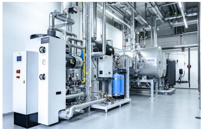
A Junior 400 TC fast steam generator from CERTUSS feeds the steam test bench in the power station at Schubert & Salzer.
