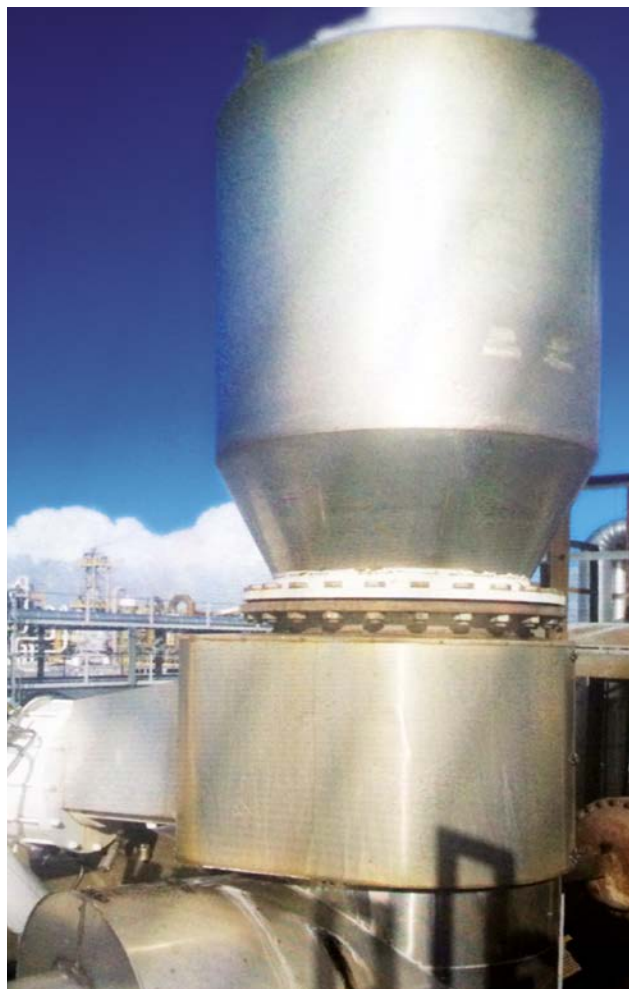
Figure 3 This insulated segment disc valve has a nominal size of 500 and is operated as an end valve with attached silencer and is operated here in a nominal size of 800.
