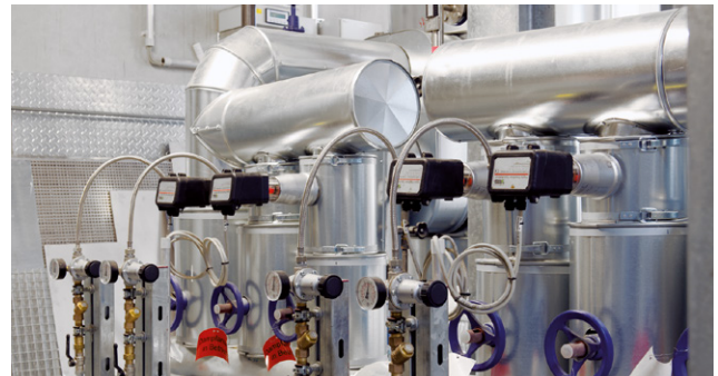
Two sliding gate valves, operated in parallel lines, secure precise condensate control for an optimum efficiency of the heat condensers.
