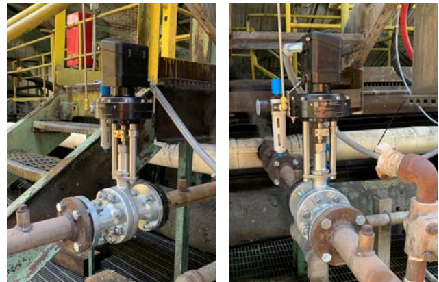
The sliding gate valve Type 8621 with flanged connection in use on the steam line at U.S. Vanadium. The overall length corresponds to that of a globe valve of the same nominal size.
